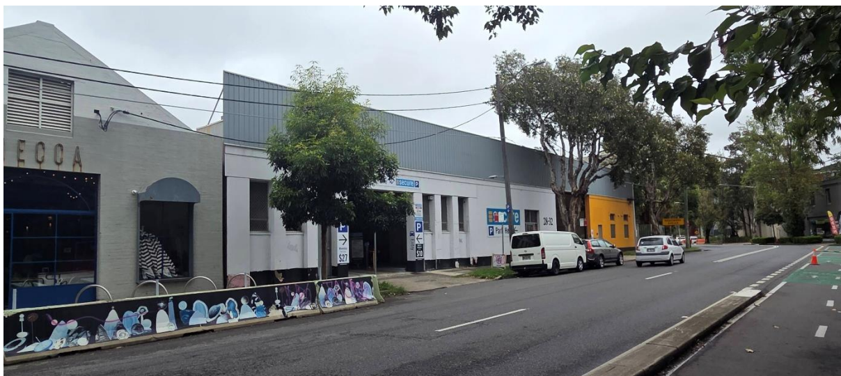
Figure 6: Western adjoining site at 28-32 Bourke Road
